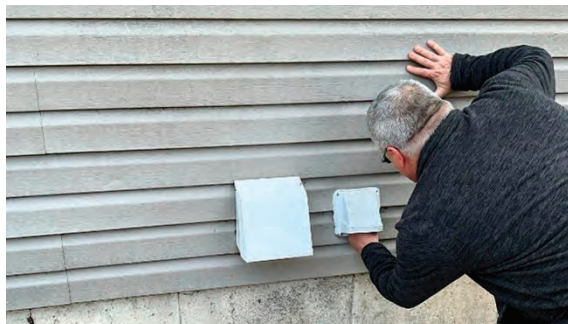
Greg Smith performing a housing inspection
